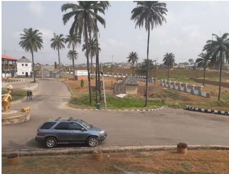
Figure 10. Absence of speed of breakers at Ife Grand Resort
