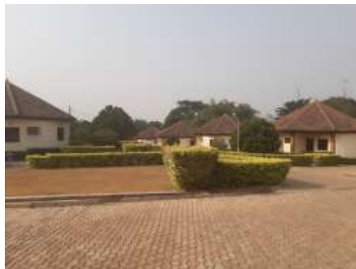
Figure 3. Access control feature at Zenababs Half Moon Resort
