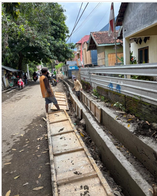
Figure 2. Formwork removal
