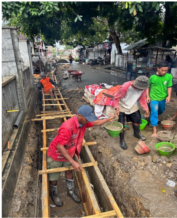
Figure 1. Drainage channel installation
