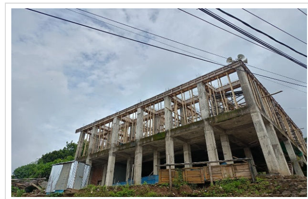
Figure 2. Condition of Reinforced-Concrete column work at the Nurul Yaqin Mosque
